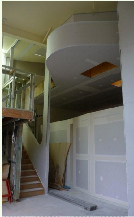
2 Pasterboard before the paint
