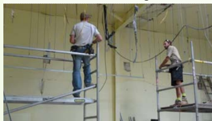
4 Suspending the ceiling supports
