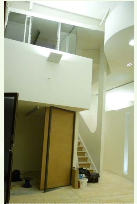
3 Paint, lights, ply ready for boards
