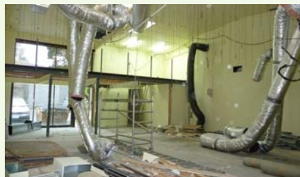
3 Demo and Aircon ducting
